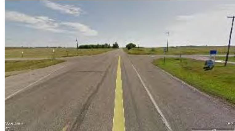
Poorly lit intersection at intersection of MNTH 200 and CSAH 3
