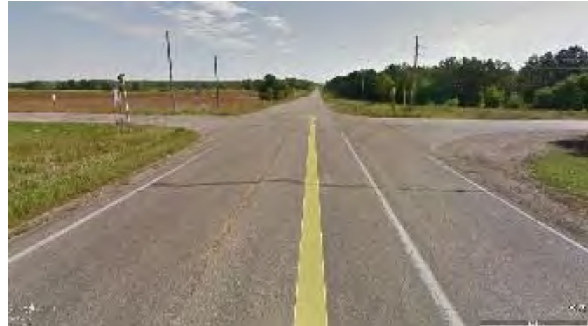
Poorly lit intersection at intersection of MNTH 200 and CSAH 4
