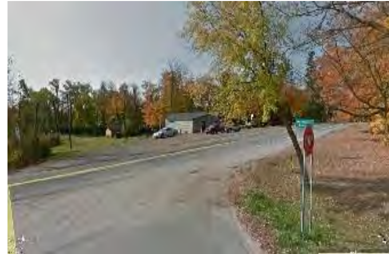
Intersection site distance issues MNTH 200/Clearwater CSAH 7
