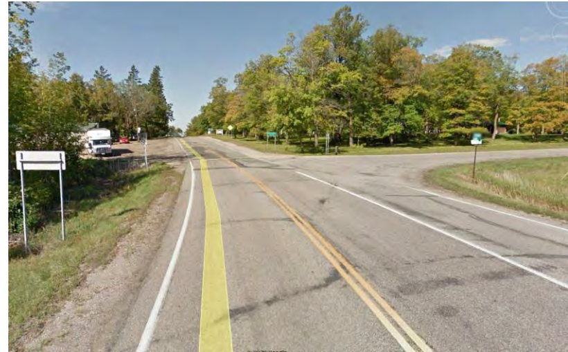
Poorly lit intersection MNTH 200/Clearwater CSAH 7
