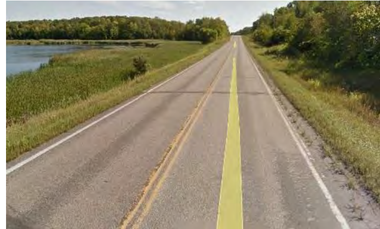
Steep ditch inslope near Goodwin Lake
