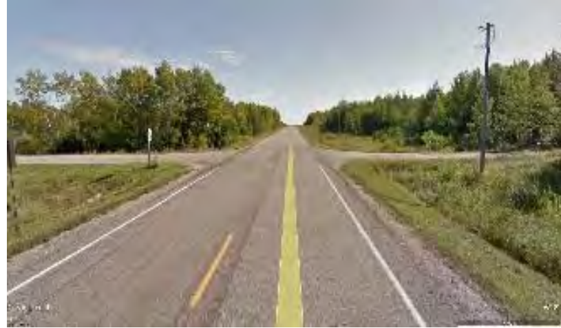
Poorly lit intersection MNTH 200/ Auginaush Road
