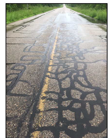
E: Extensive chip sealing on Blair Road shows need for pavement rehabilitation
